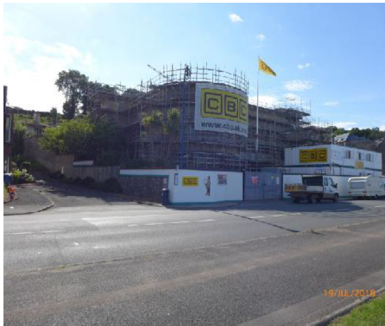
South and East Elevations
