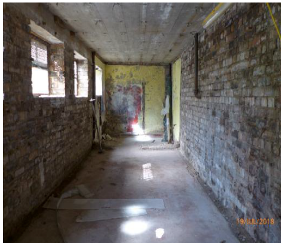
Upper GF - Toilets at Main Stair Half Landing
