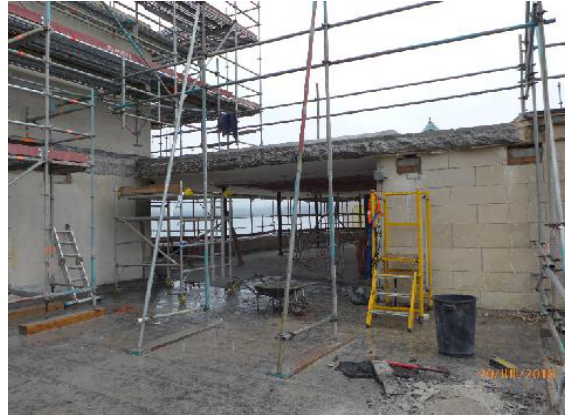
Removal of the overhang in progress.
