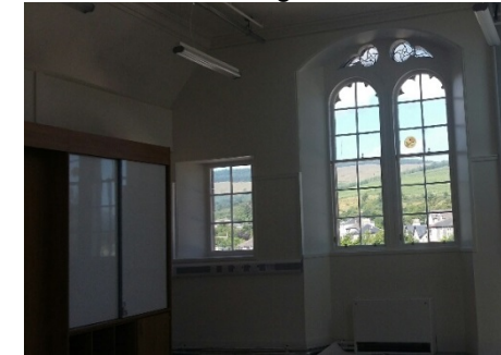
Refurbished original windows
