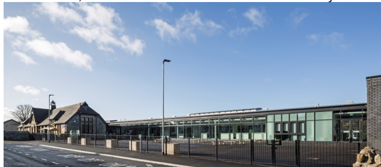
Front elevation of the new Kirn Primary School
