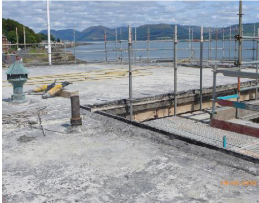
Existing roof finishes previously removed
