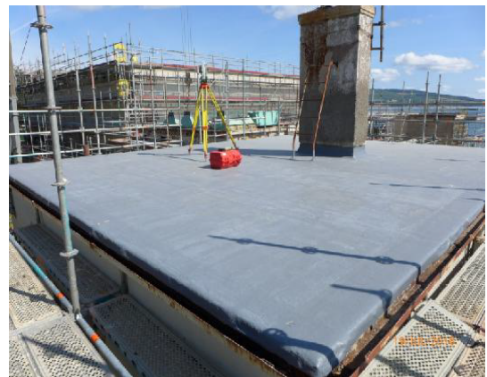
East & West Elevations – temporary protection in place over the new roof membrane.
