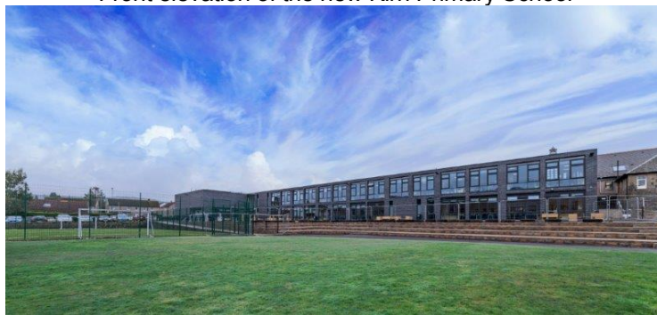
Rear elevation of the new Kirn Primary School
