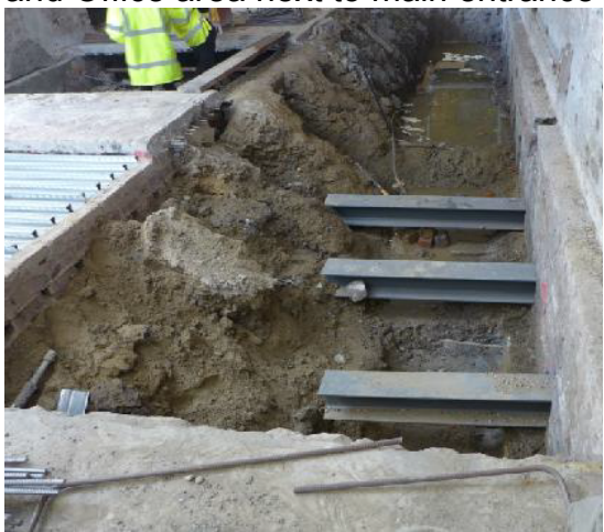
Lower Ground Floor – Main entrance Foyer / Circulation area – steel beam installation through the wall and into Undercroft area for works to strengthen the existing west wall.
