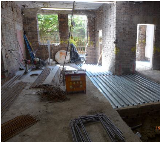
Lower Ground Floor – Reinstatement of floor removed to the existing Store and Office area next to main entrance Foyer / Circulation area in progress.
