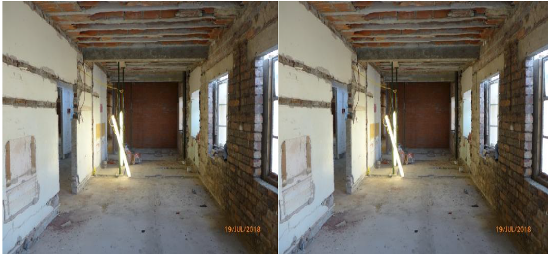
Upper Ground Floor – Back Stage Area.
