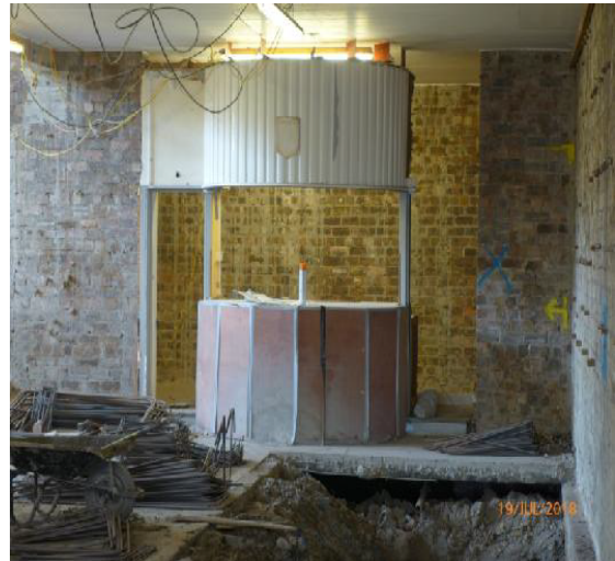
Lower GF – Section of Protection to the Reception Desk has come away, no works ongoing at this area at present
