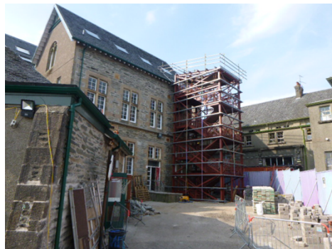
Temporary Escape Stair Installation
