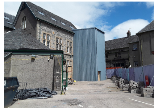
Complete Temporary Escape Stair
