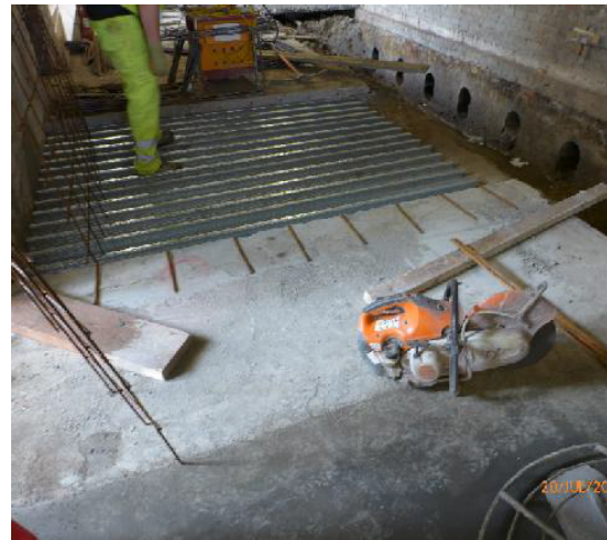
Lower Ground Floor – Reinstatement of floor removed to the existing Store and Office area next to main entrance Foyer / Circulation area in progress.
