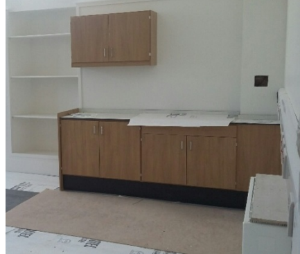
2 nd Floor Classroom Wet Area
