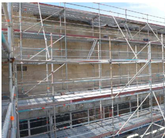
East Elevation – Pavillion sign elevation (sign previously removed)
