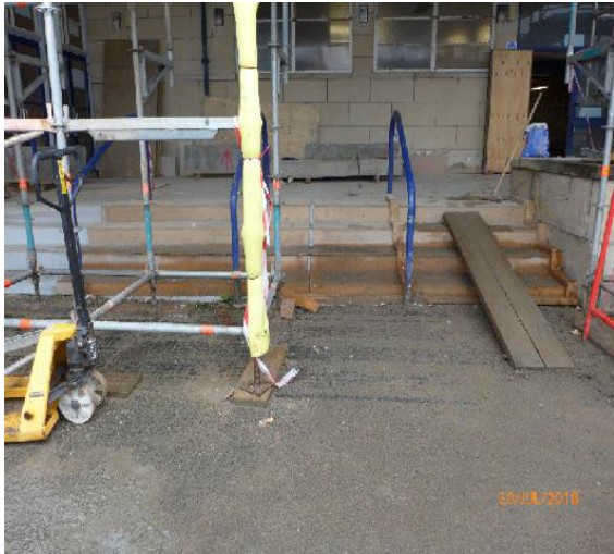
Front Entrance Steps – Protection Maintained.
