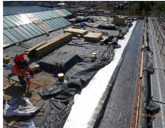
East & West Elevations – temporary protection in place over the new roof membrane.
