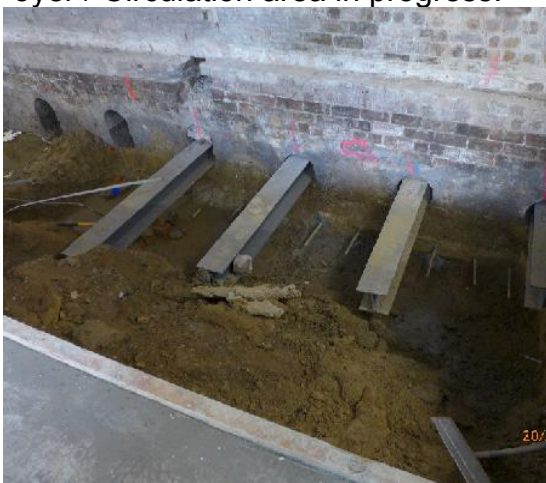
Lower Ground Floor – Main entrance Foyer / Circulation area – steel beam installation through the wall and into Undercroft area for works to strengthen the existing west wall.
