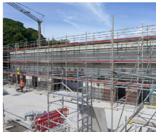
Southern Terrace wall.
