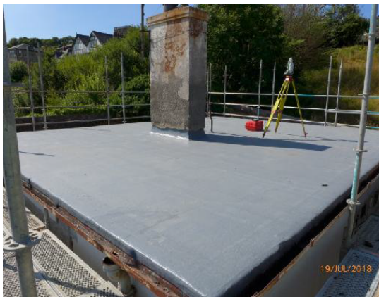
New roof covering installed.
