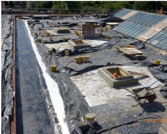
East & West Elevations – temporary protection in place over the new roof membrane.
